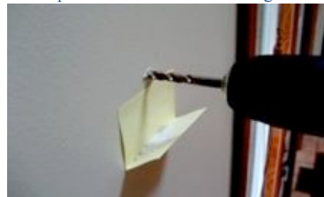
Use a post it note to catch drilling debris.
