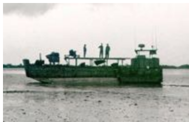
Above: A port side view of the Nha Be HSSC. Note the gap between the edge of the top deck with the M40A1 recoilless rifle and the twin .50 gun tub. [Photo: Ron Allen]
