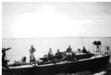
Above: A Mk 4 LCPL as hastily modified by members of ST-1. Some guns lack armored shields to protect the gunners and the crew is much too exposed. Whether it was used on operations is not known. [Photo: Chuck LeMoynes]
